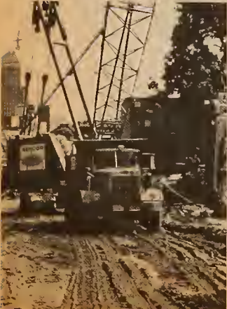
Step 2: Excavation of Trenches with Special Clamshell Equipment.
